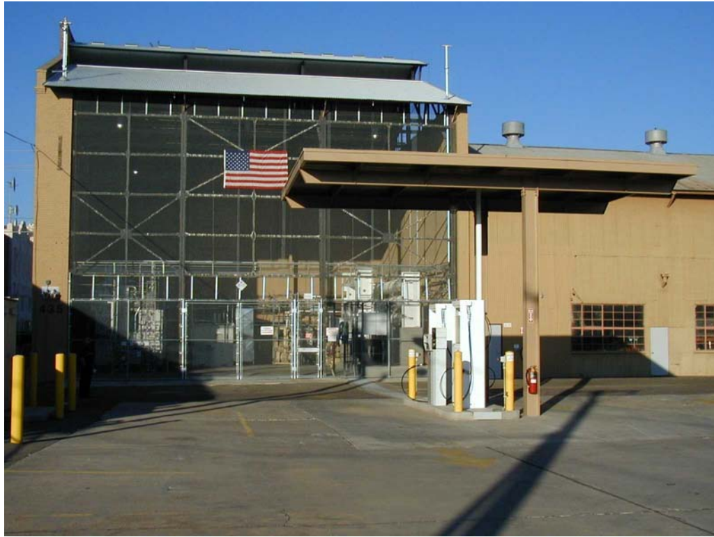
Figure 1.2. East Side of the APS Alternative Fuel Pilot Plant.
