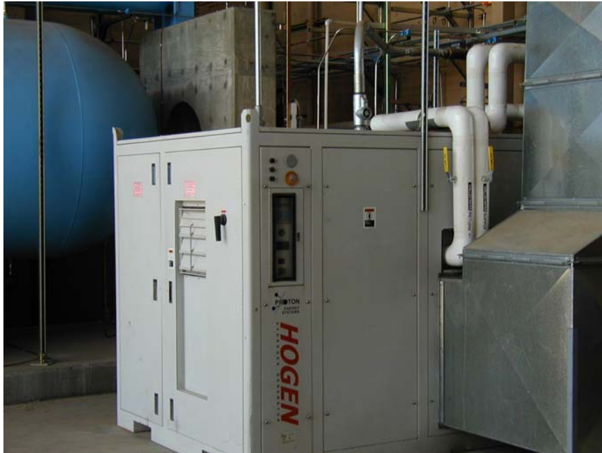
Figure 2-1. HOGEN 300 proton exchange system.
